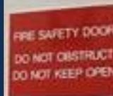
Fire resistant doorsets, commonly called fire doors, are an integral component of fire protection in buildings and classified as passive fire protection systems. They are installed in walls constructed as fire barriers. Each fire door and the wall housing it, have a fire rating known as a fire resistant level.
