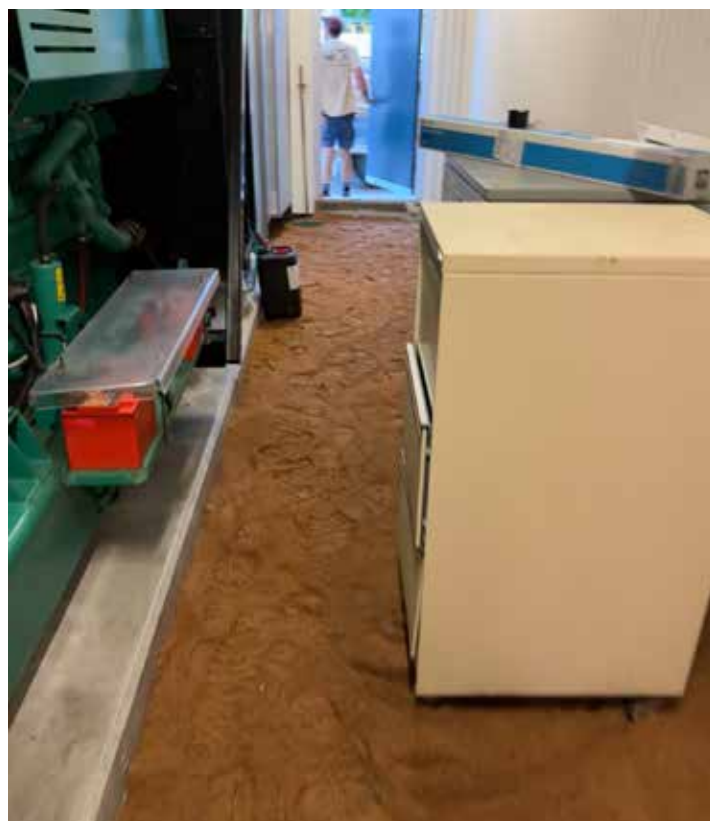
Firefighters covered the floor in sand to soak up the remaining diesel.
