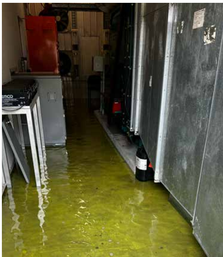
About 1500 litres of diesel leaked into the generator room.
